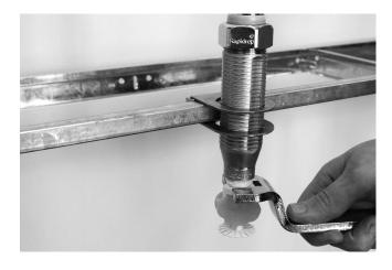
When installing the sprinkler head with a two piece escutcheon, the inner piece should be mounted on the thread of the sprinkler head before attaching to the reducer.
